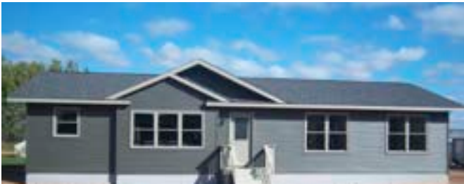
BOX BAY TO FLOOR OUTSIDE
