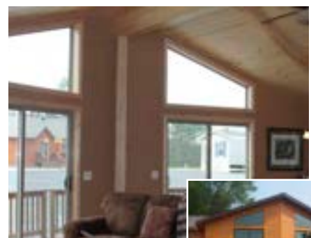
4/12 PARALLEL CHORD WITH KNOTTY PINE CEILING & PINE BOX BEAMS (Interior)
