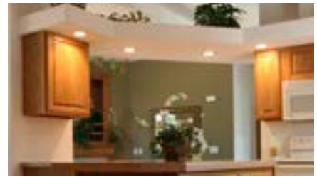
Extended Hanging Soffit Above Cabinets
